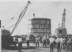
THE TWO mobile cranes were put to good use as they slid the forty-five-ton storage tank off the barge near Gerard Dock. E DOS grua móvil a haci bon trabao habando e tanki di cuarenta y cinco ton for di e lancha na Gerard pier.
